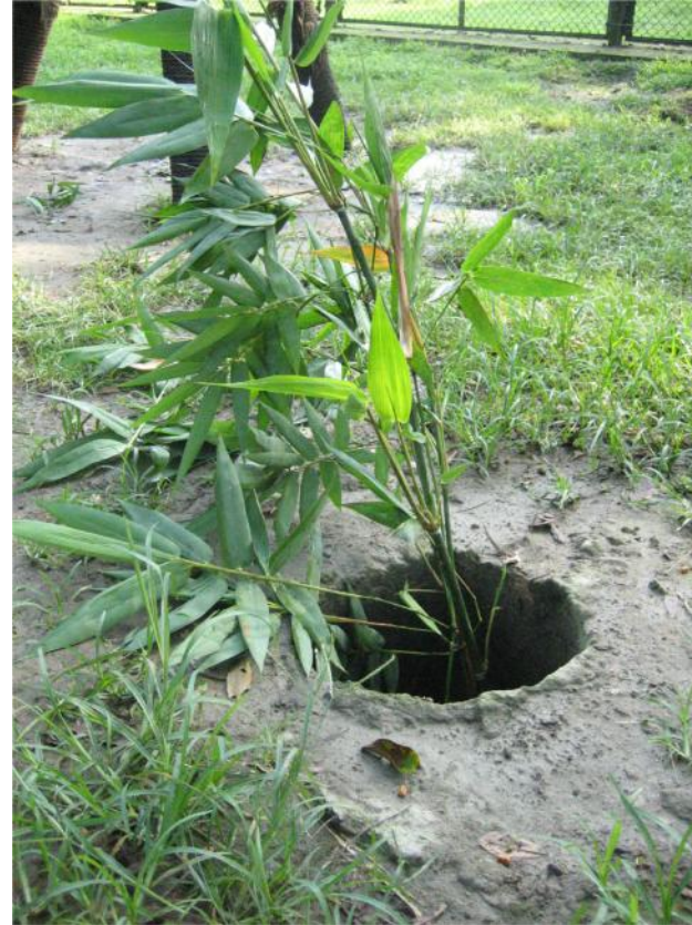
Concrete tunnel vertical
