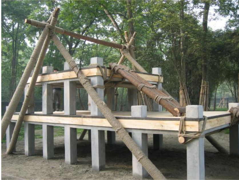
A-frame platform (with concrete support post)
