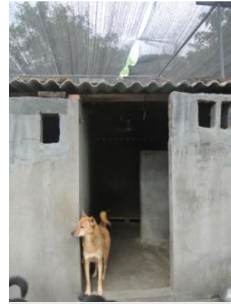
The top of the shelter is now fixed
